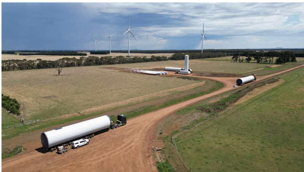
Delivery of the last load
